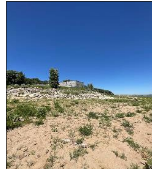
Cannon Ball intake with exposed pipe (facing northwest)
